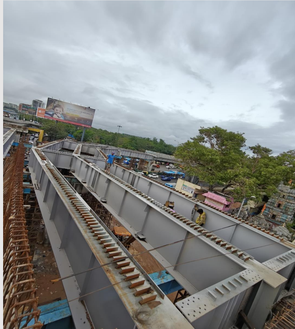
TB19-TB20, TB20-TB21, TB21-TB22 Spans Bracing Fixing Work
