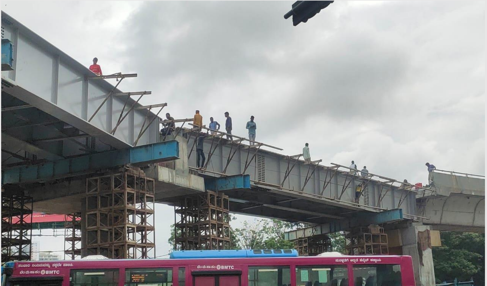
TB21-TB22 & TB22-KP6 Deck Slab Shuttering Work
