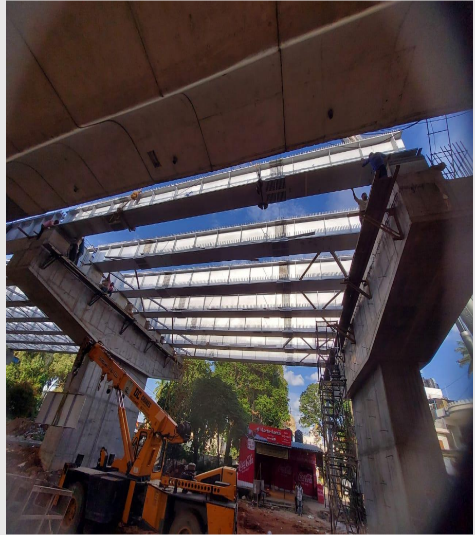
AB14-AB15 Span Erection Work
