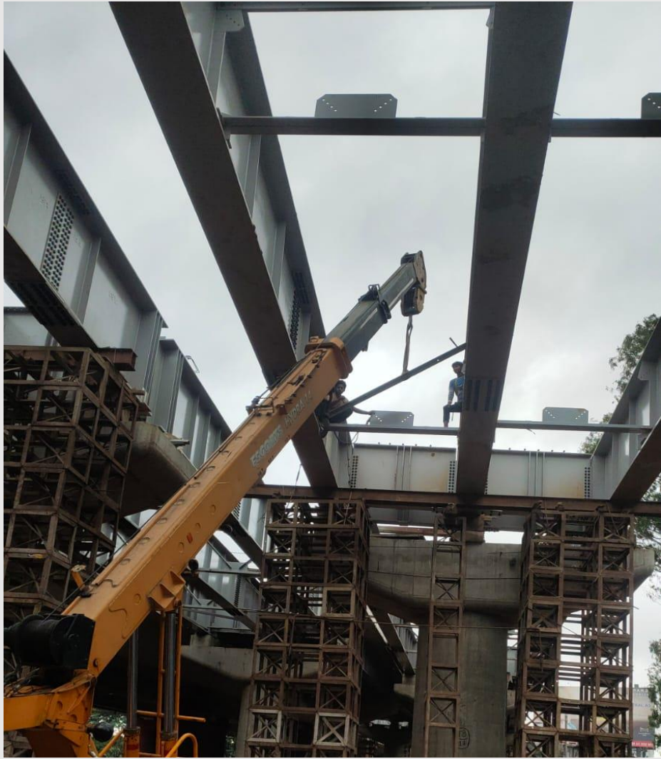
AB16-TB17 Span Bracing Fixing Work
