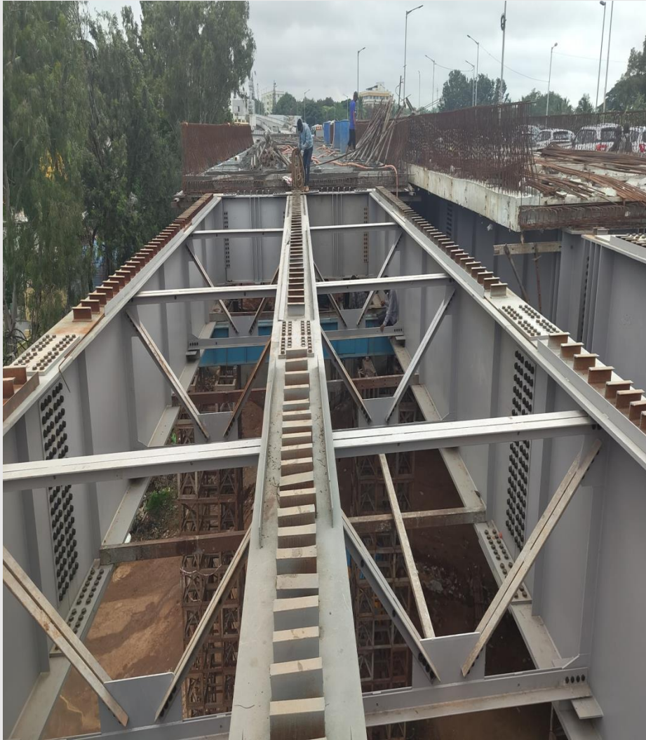
TB19-TB20, TB20-TB21, TB21-TB22 Spans Bracing Fixing Work
